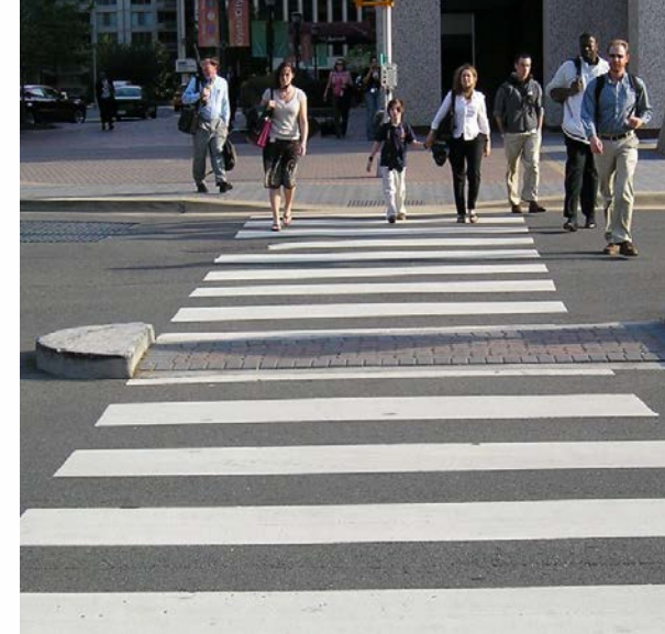
High Visibility Crosswalk Striping City Standard Crosswalk Treatment
